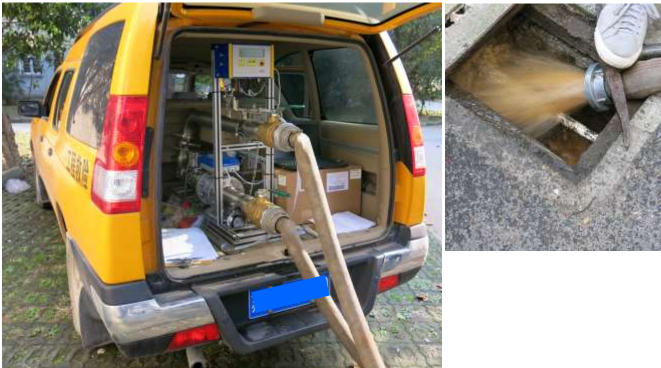
Figure 3: Flushing device FlushInspect installed in a up pickup car of the water supplier (left) and mobilization of deposits due to the increase of the flow velocity by the flushing
